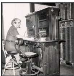
ENA CHAPMAN AT THE SWITCHBOARD. THE PHONE SYSTEM'S DISTRIBUTION FRAME IS IN THE BACK.
